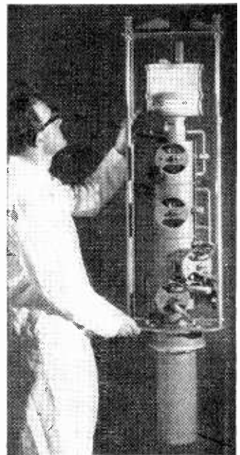
25 kW klystron from S.T.C.
